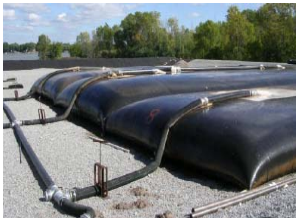
Fox River OU1 2004 Pilot Test geotubes
